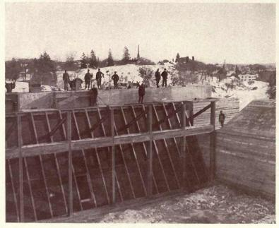
WO views of the interior of the forebay above the power house with some detail of the racks and the temporary spillway. The first picture is looking up the river through the coarse racks. The fine racks and the penstock gates are on the right of the picture.
